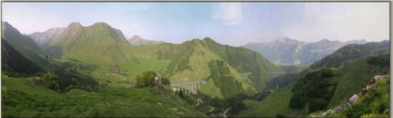
15 years after completion (2040)
