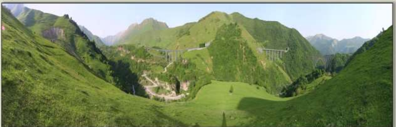
15 years after completion (2040)
