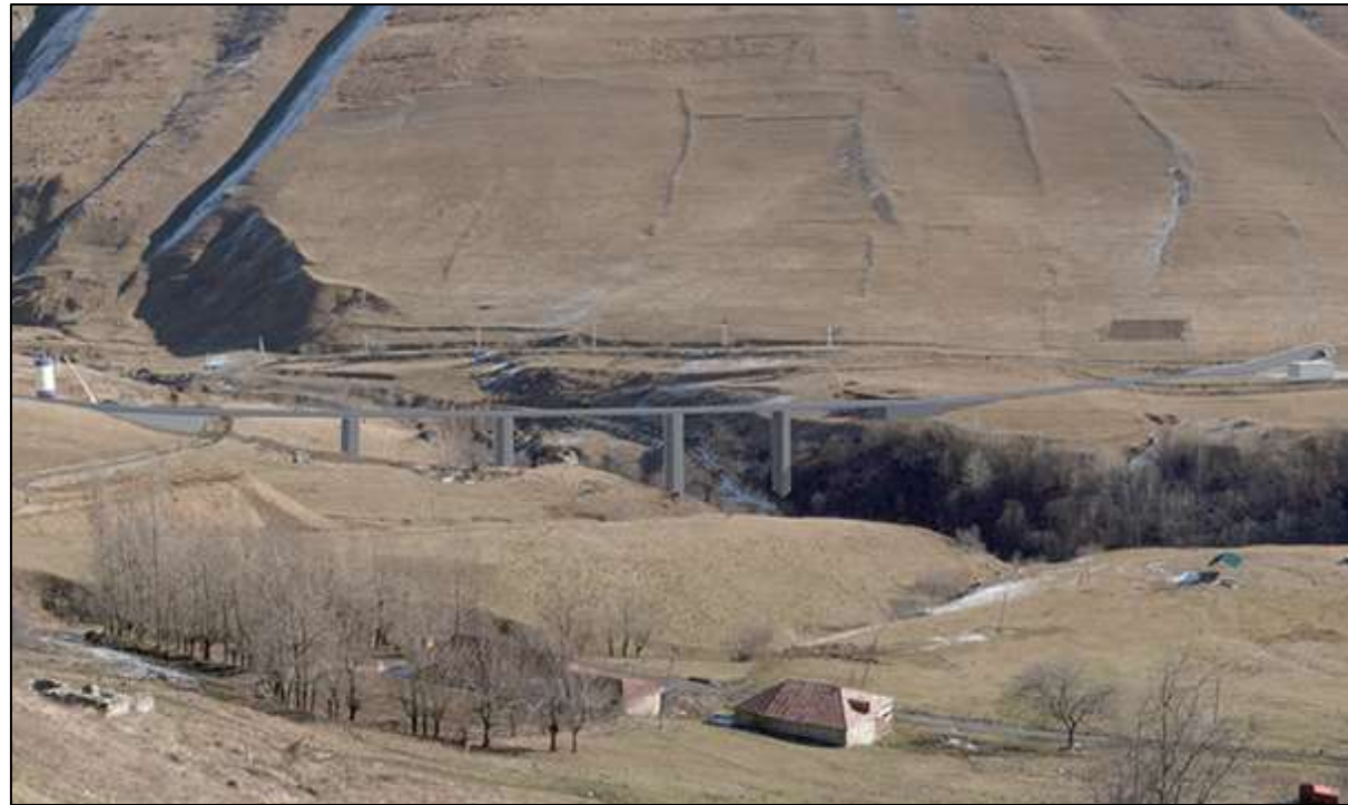
Render of the view west to east across Khada Valley towards Bridge 6
