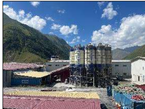
Lot 1: Kobi batching plant
