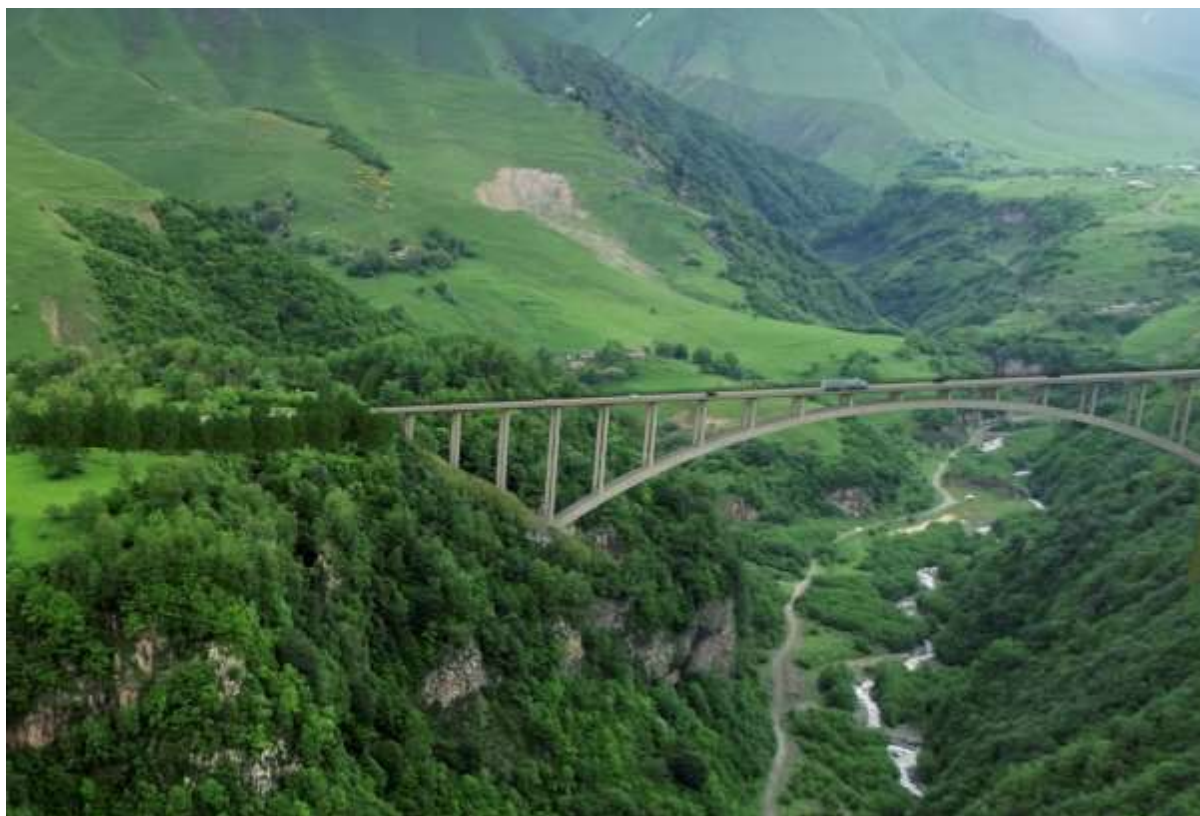
Figure 4: Arch Bridge (Bridge #3)
